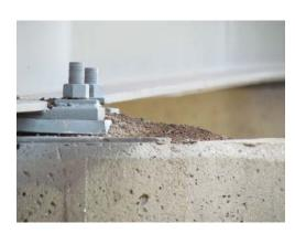
Photo 5: Guano deposit on pier, obscuring structural features.
